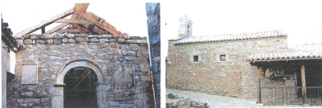
Holy Trinity chapel pictured before and after restoration
