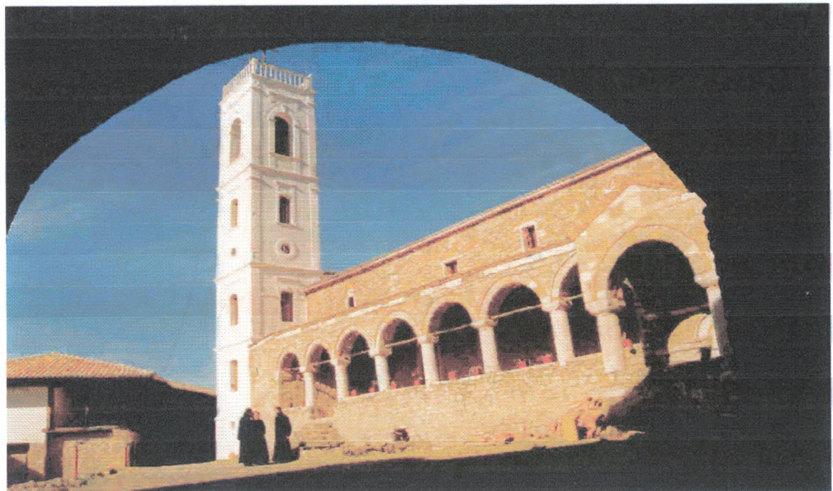
The Monastery of Ardenicë, Myzeqe. The catholicon during and after the 1996-1999 restoration interventions.
