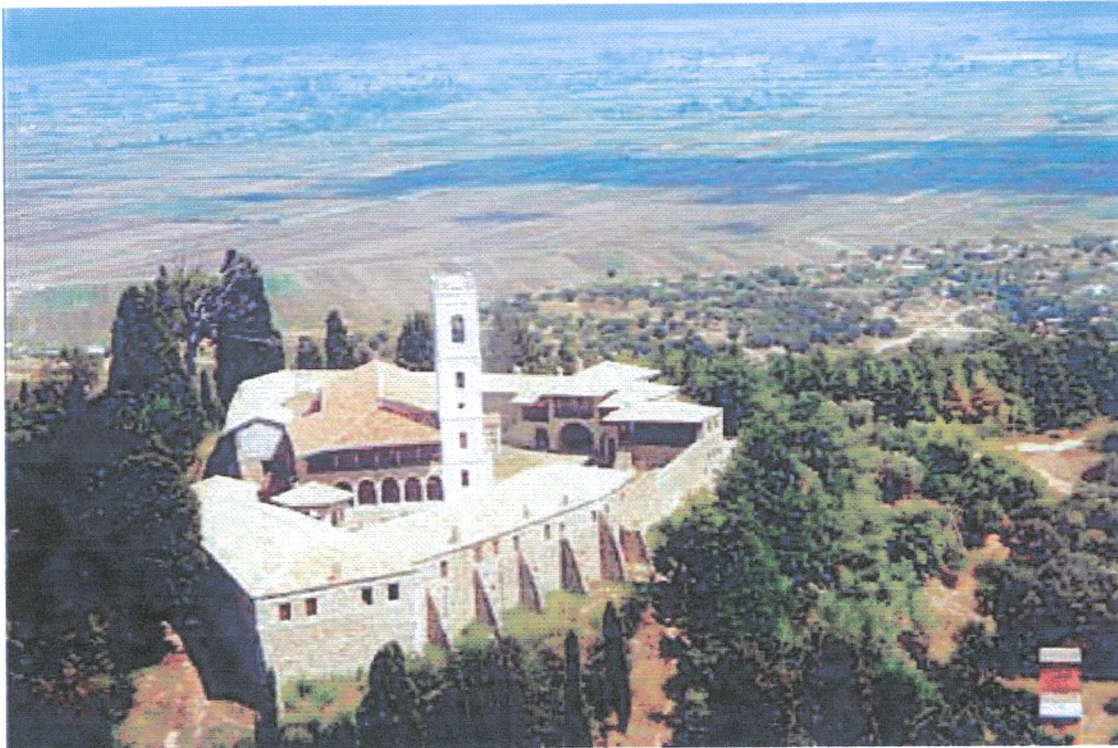
General view of the monastery from the W.
