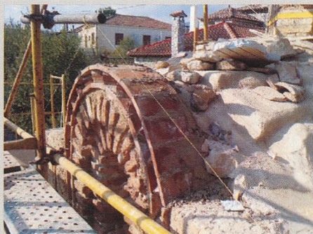
The monument during the restoration works
