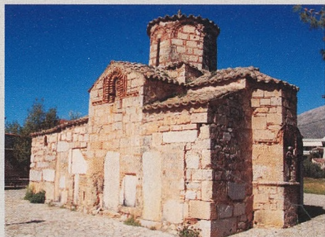
The church before the restoration
