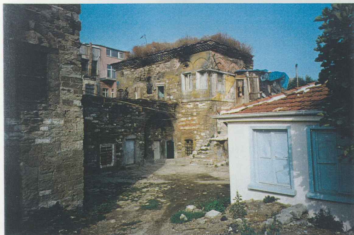
Ill.5 View of the inner courtyard between the buildings no 2, no 3 and the church from southeast.
