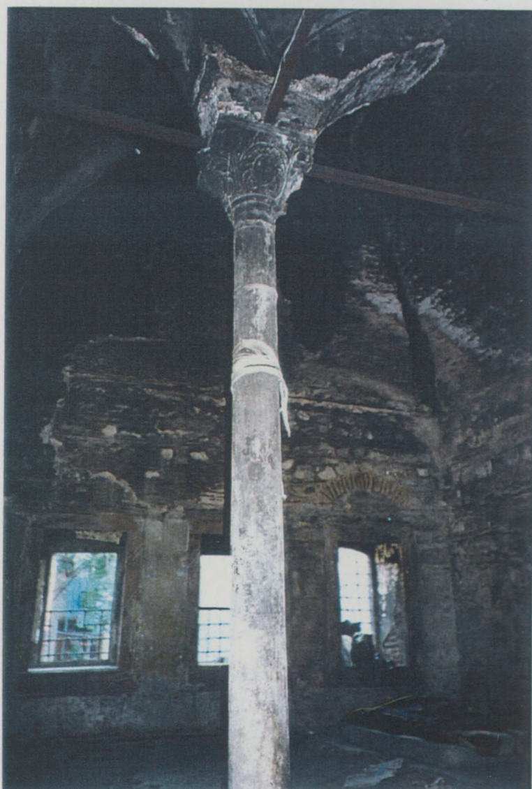
Ill. 13 View of the interior of the mansion no 6.
