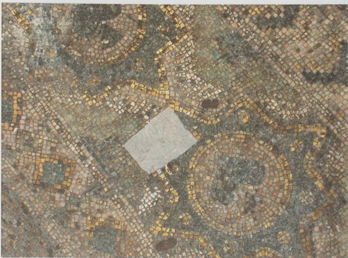
Metallic clamps in the ceiling's mosaic.
