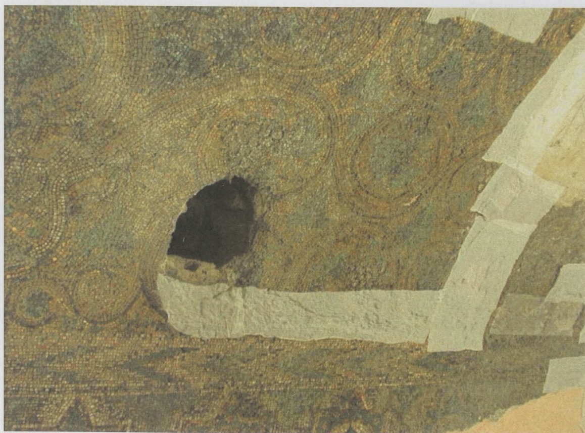
Opening for an ancient conduit in the ceiling.
