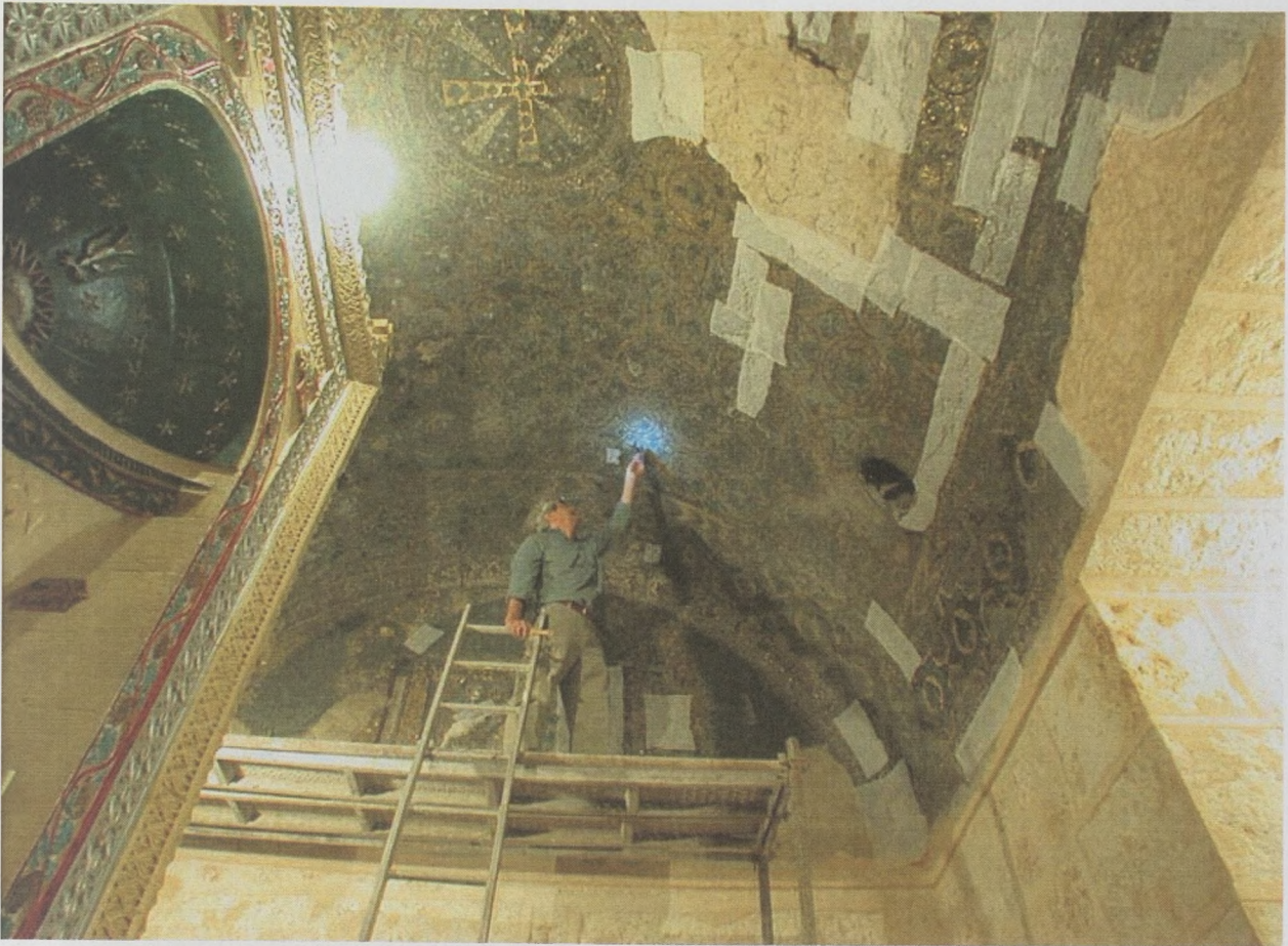
Using a small scaffold, we were able to examine part of the mosaic.
