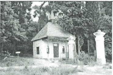
Photo No 7: Guardhouse of the Internal gate
