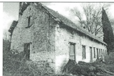
Photo No 4: Building for the workers
