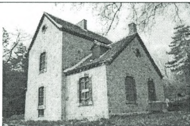
Photo No 10: Building for the Officers of the Guard
